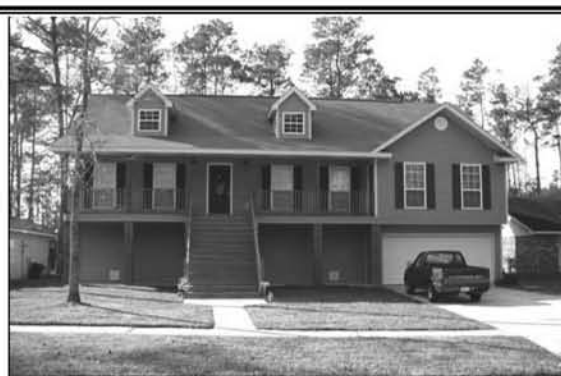
This repetitive loss house was elevated with help from a FEMA grant.
