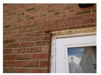
**Cracked Brick and Rusted Lintel**
