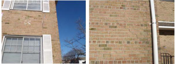
Photo B: Vertical crack at corner Bldg 9
