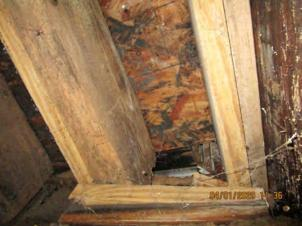
Rotted and Missing Wood Sill in Crawl Space
