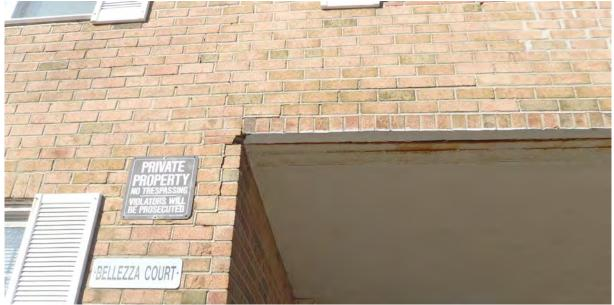
Photo J: Crushed brick and rusted lintel over carport
