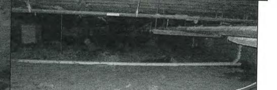
Photo E - Improperly Supported Piping
