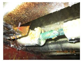
Leaking Water Pipe in Crawl Space
