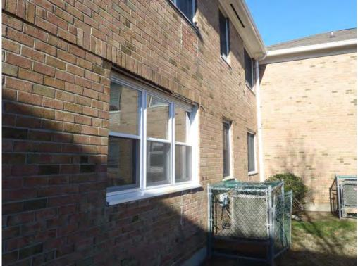
Photo A: Continuous horizontal crack and rusted lintel at Bldg 9 west courtyard wall
