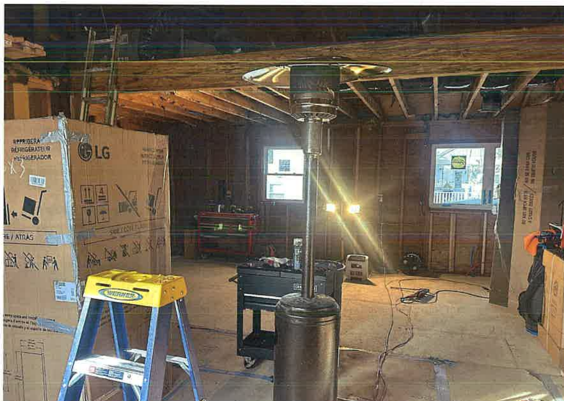
Image shows the beam that replaced the wall between the living room and kitchen. Beam has been permitted and is shown in the architectural plans as an open concept space.
